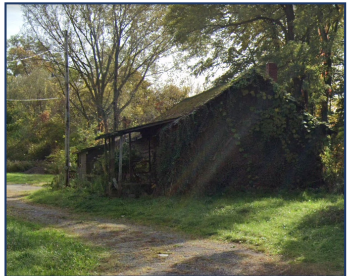
The old Log Cabin just south of the Route 20 underpass prior to demolition. In the Winter 2023 issue of The Harbor View newsletter, Jane Ingold wrote an article highlighting stories and memories collected from other community members. Credit: Google Maps.
