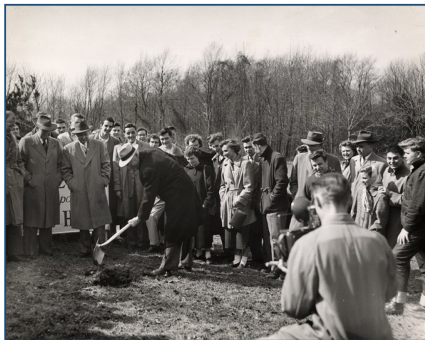
The 1952 groundbreaking for Erie Hall. Photograph courtesy of Behrend Archives.
